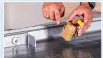
Limit Switch Installation
